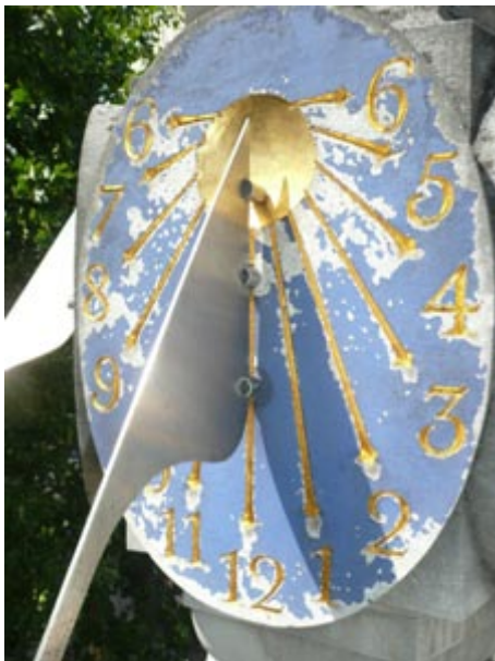
Damaged South Dial.
