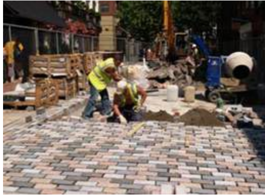
2006 Monmouth St sett laying.
